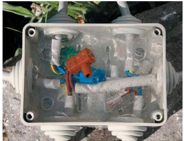
Fill the entire void all the way to the top, ensuring there are no air bubbles or gaps when component is closed. Gel will then smooth out to fill the entire space, so make sure that enough gel is used, if not enough add more.
