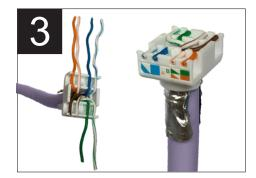
Flush cut the extra conductor length using wire cutters so it is flat to the edge of the termination cap.
